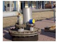
4300 locations that manufacture refined chemicals from petroleum and hydrocarbon based material. Chemical plants are hazardous environments that require explosion proof or intrinsically safe certified instrumentation. Here, an EchoSafe ultrasonic level transmitter is installed on the man-way cover of a below grade wastewater storage tank. Our patented digital signal processing features an industry leading 3" beam width that enables installation next to their 6" suction pipe.
